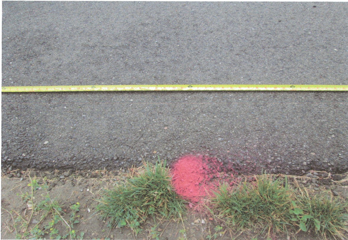
Boundaries for pavers marked by Pleasant Prairie on existing asphalt driveway.
